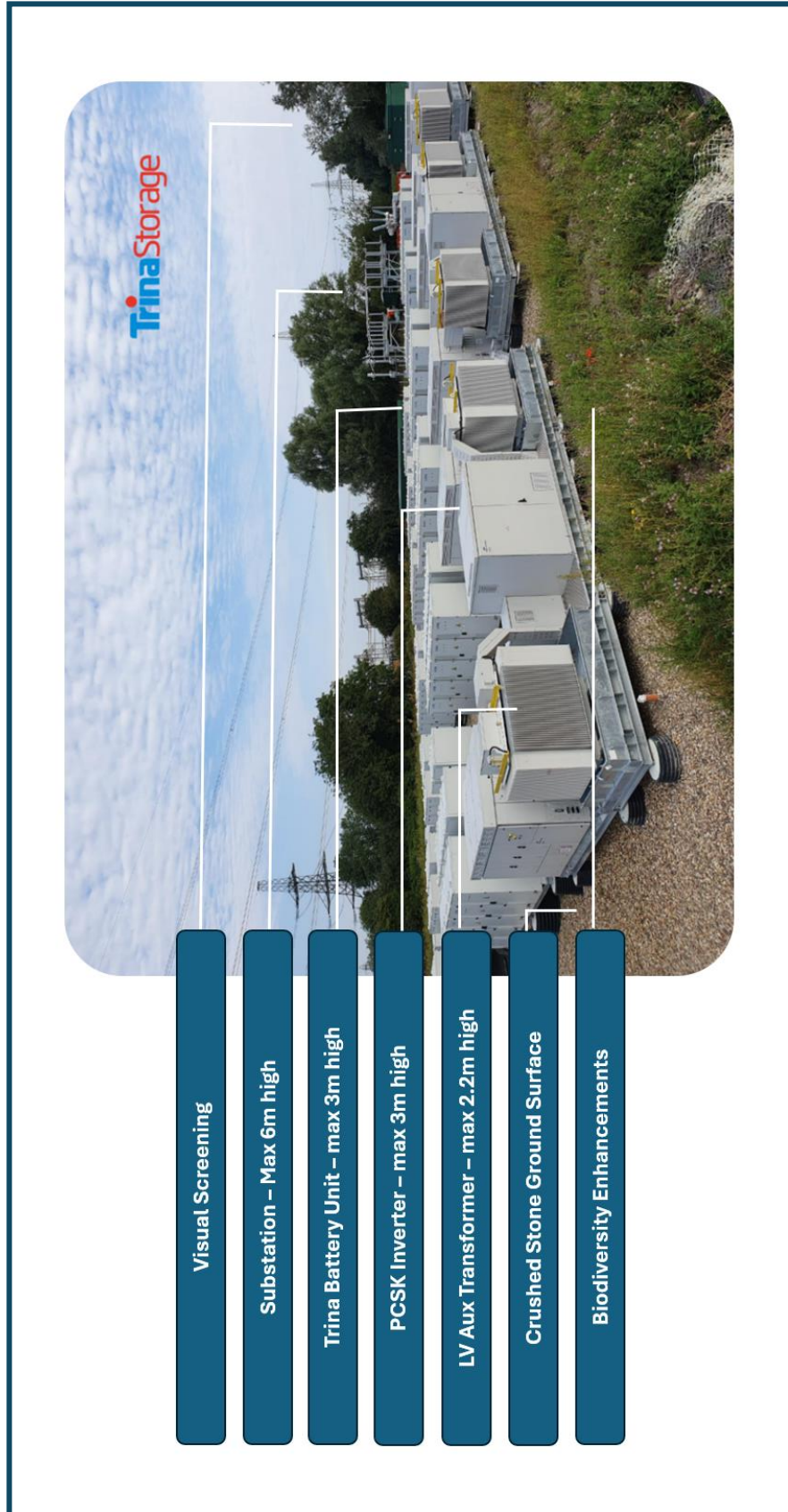
Figure 1: A photo illustrating the typical design of a BESS facility, such as the one proposed at Halfway House Farm
